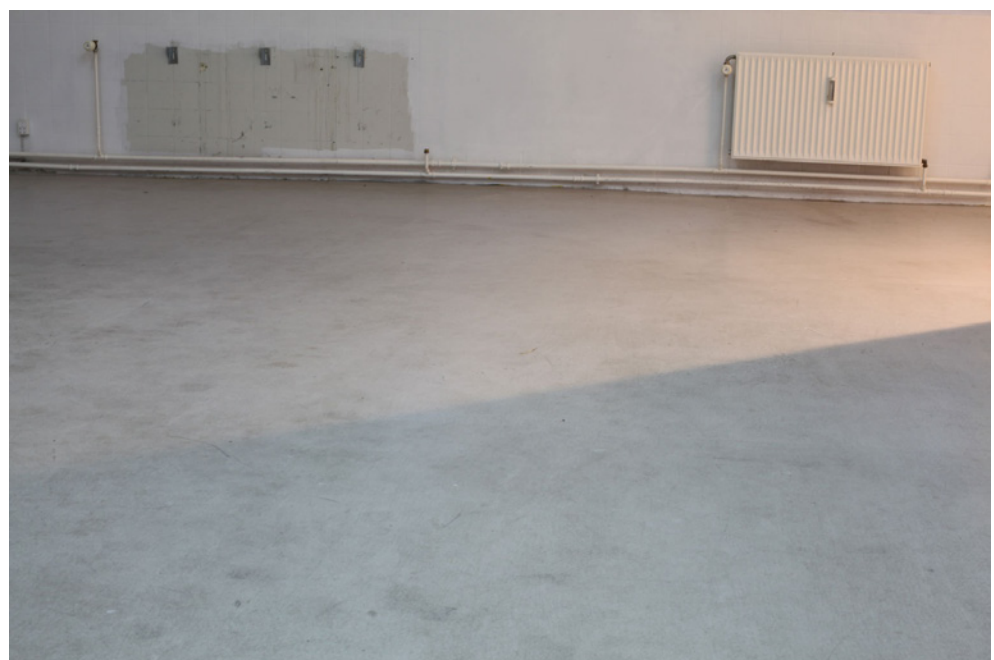
Jason Dodge, Katherine Bissell Dodge, A radiator removed from a room, 2011.
